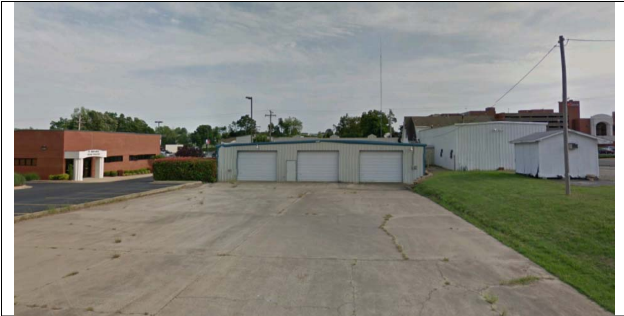
View of property looking South at rear of property.
