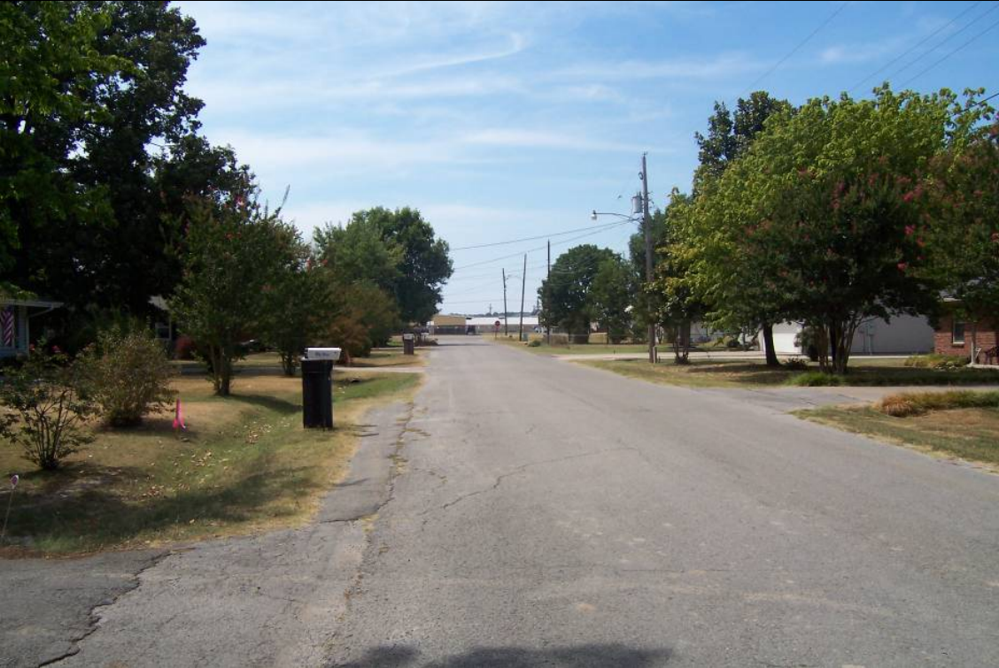
View of the site looking to the west along Sun Avenue
