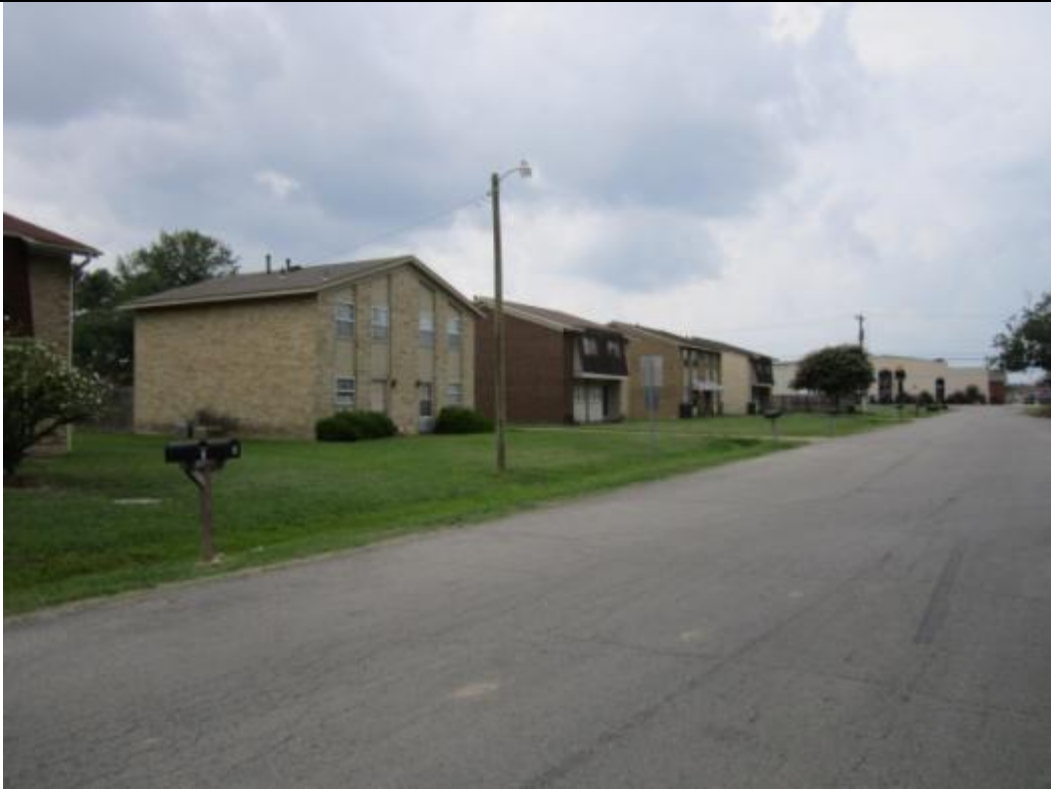
View looking west toward properties located on the south side of Fairview Drive.
