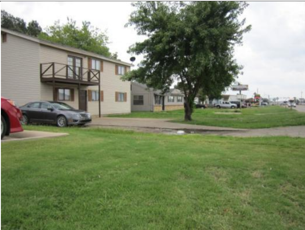
View looking south toward subject property fronting Red Wolf Blvd. from the northwest corner of subject property.
