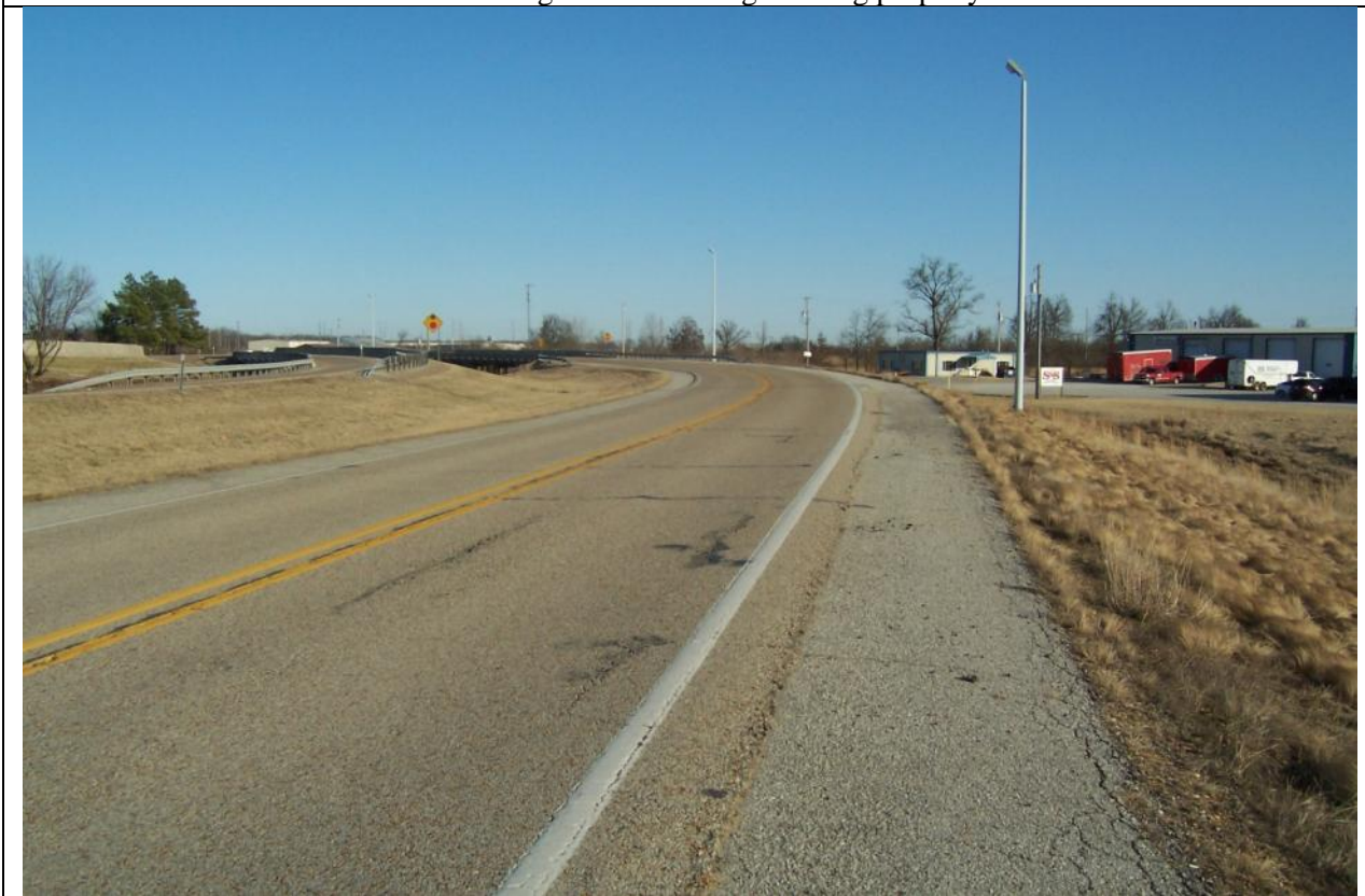
View looking southeast from subject property.
