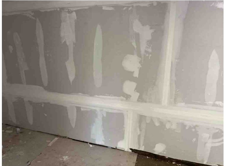
Interior of Storage Shed
