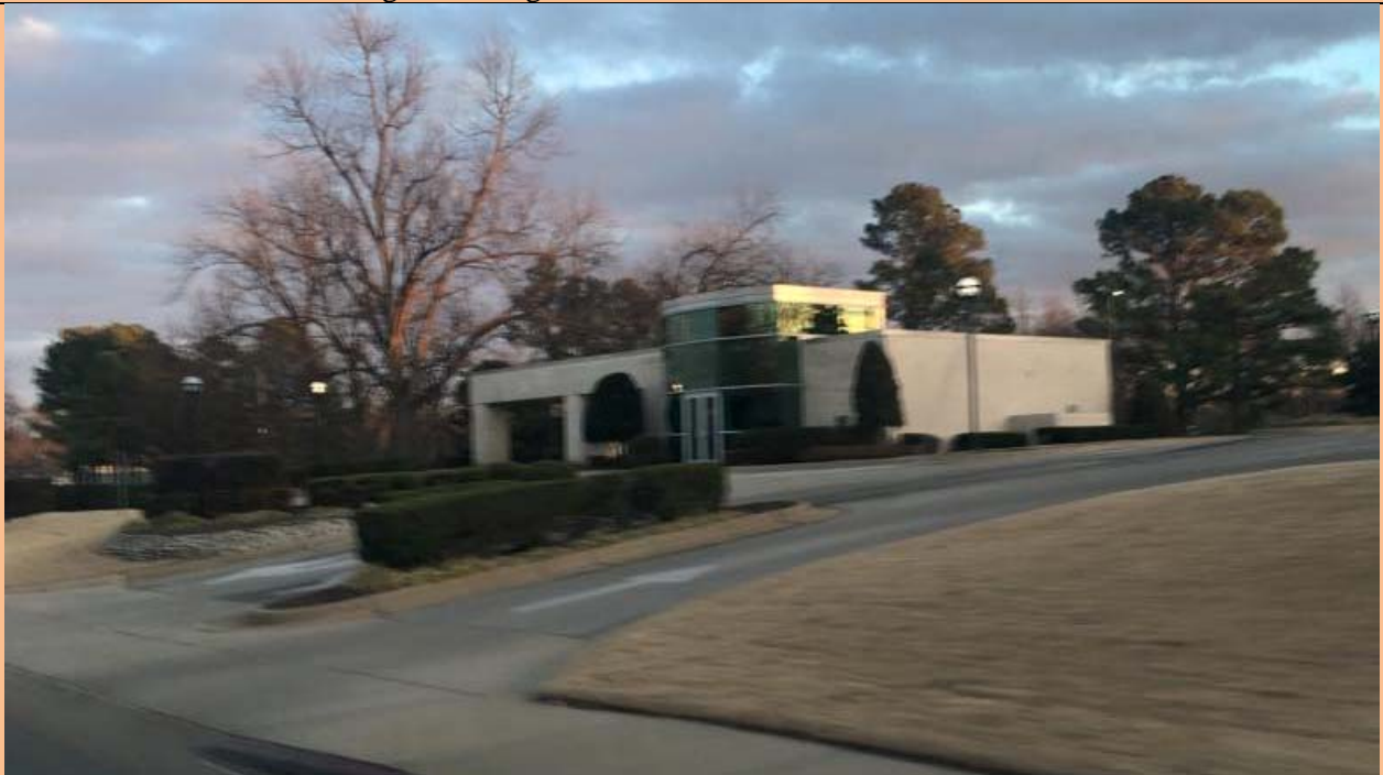
View looking Southwest at Bank, West of Site
