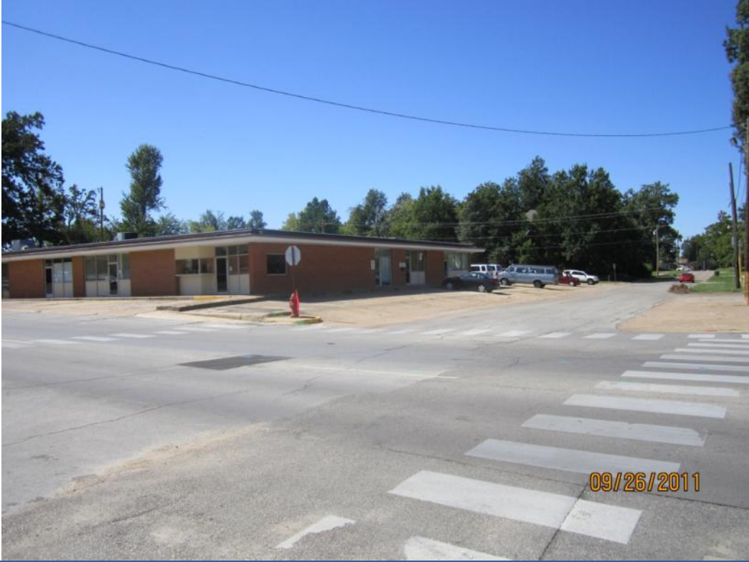
View looking West of church property.
