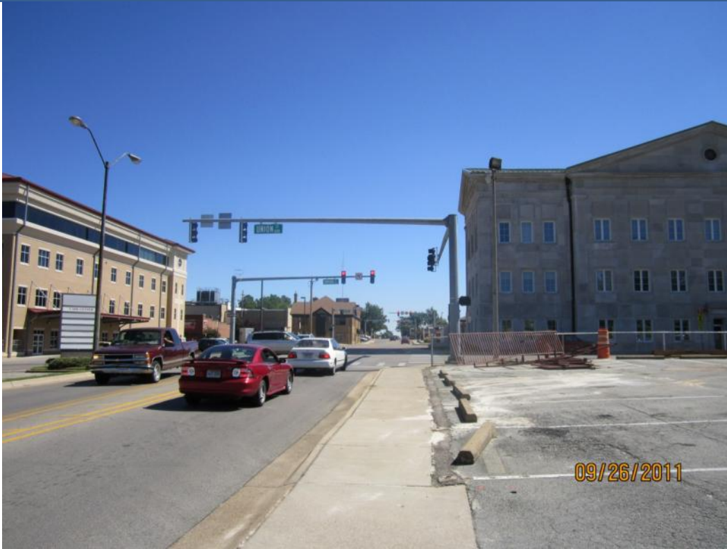
View looking East along Matthews Ave.
