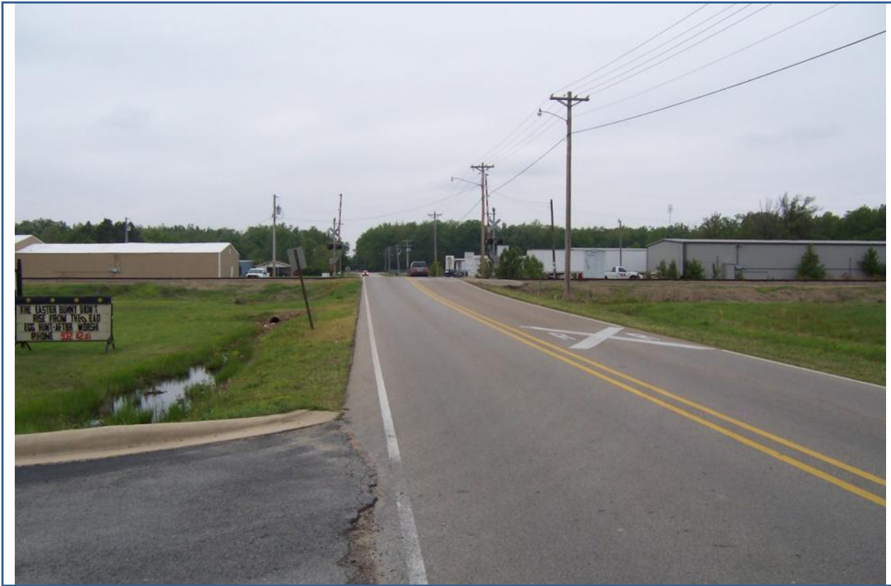
View looking West along Colony Dr of subject frontage and adjacent drive.
