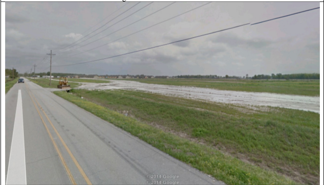
View looking Northeast on Commerce Dr., Apartments to the North of site
