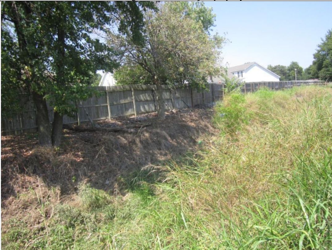
View looking North of ditch from subject property's (rear yard).
