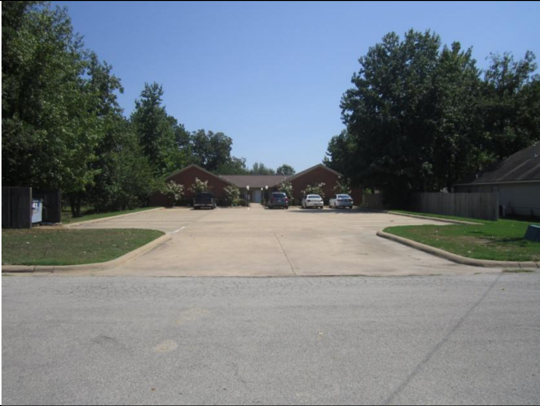
View looking Southeast of subject property.
