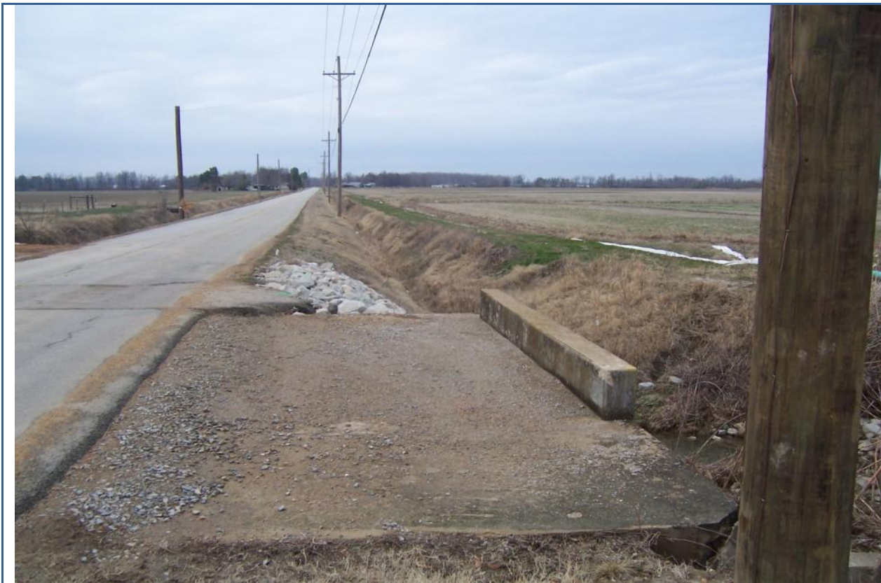
View looking North of subject property frontage and drainage ditch.
