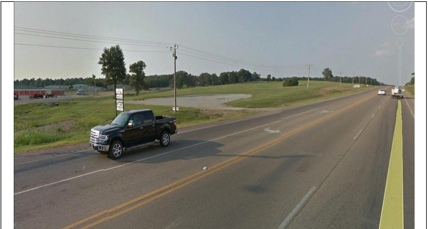
View looking Northwest of property
