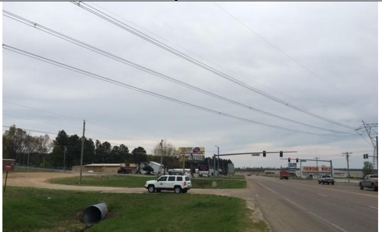
View looking South/ Site on Left
