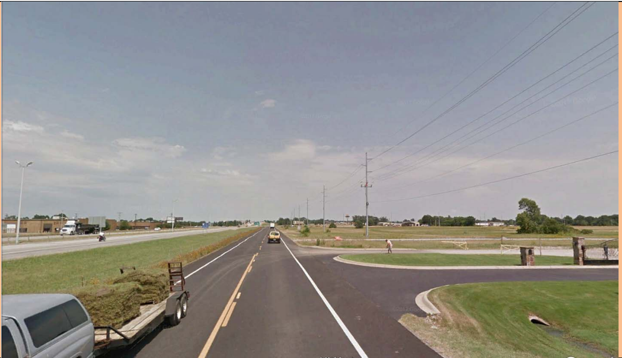
View looking East
