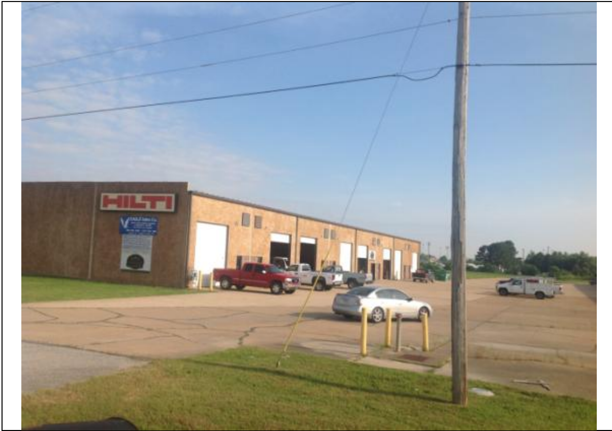
View looking north near entrance
