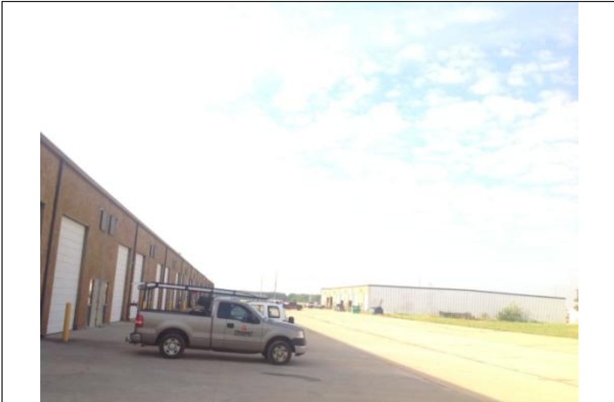
View from site looking south
