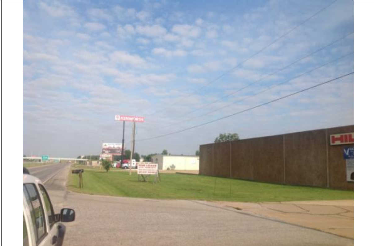
View looking East on Access road
