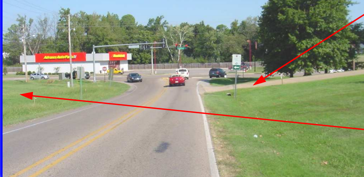
Looking north on Harrisburg Road toward Highland Drive.
