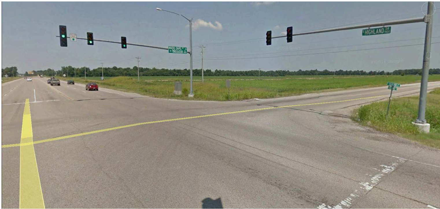
View looking from Intersection of Rogers Chapel and E. Highland towards the NW
