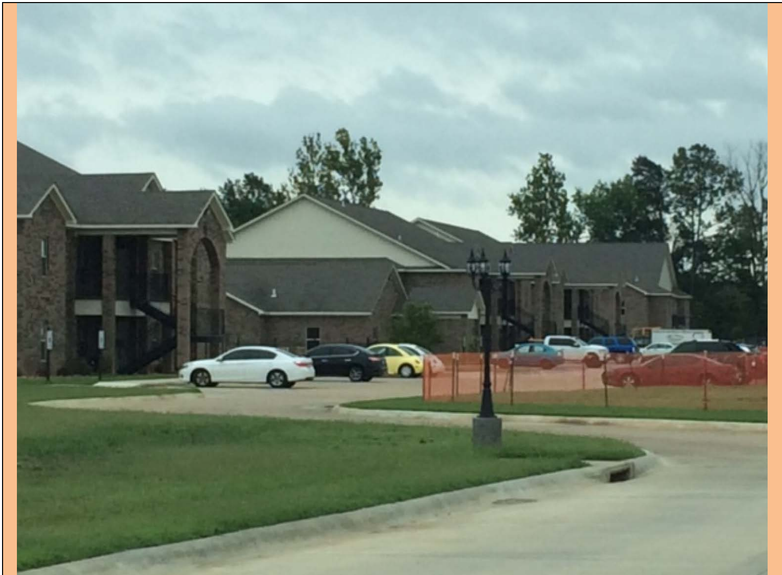
View looking Southeast toward apartments
