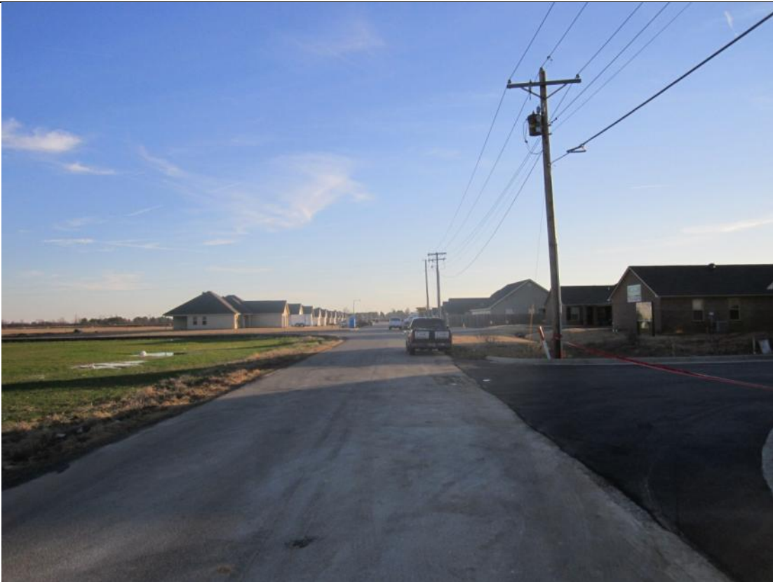
View looking South towards site along Richardson Dr.
