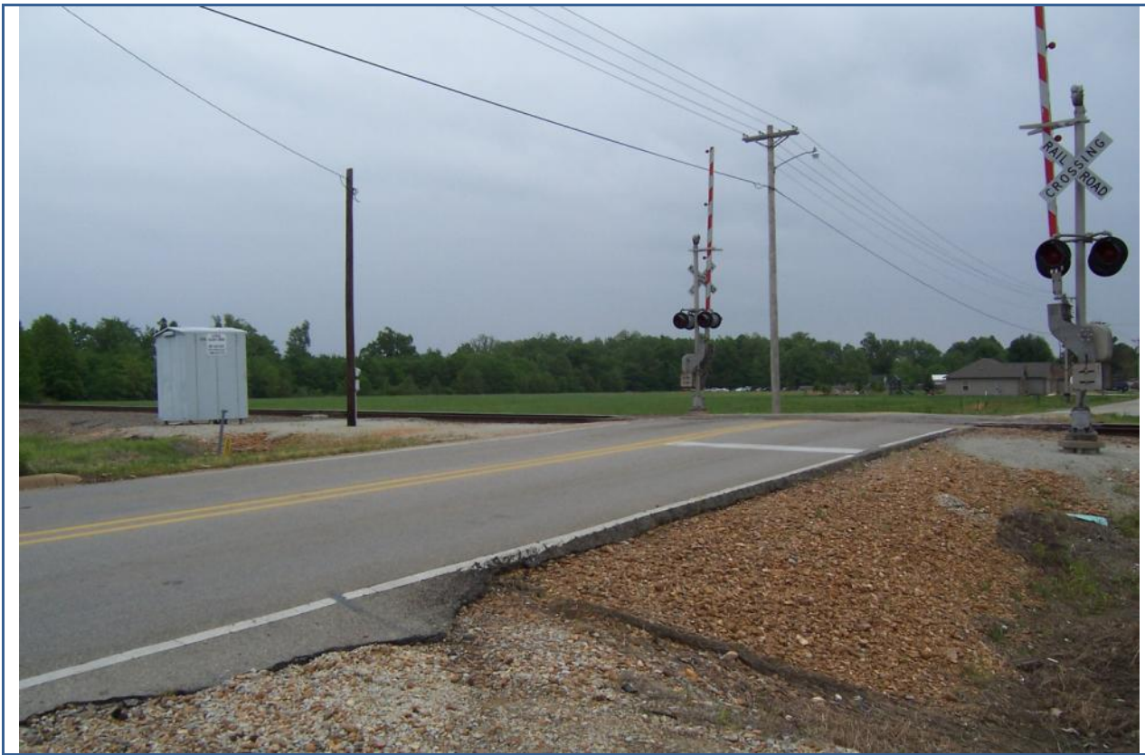
View looking Northeast towards site
