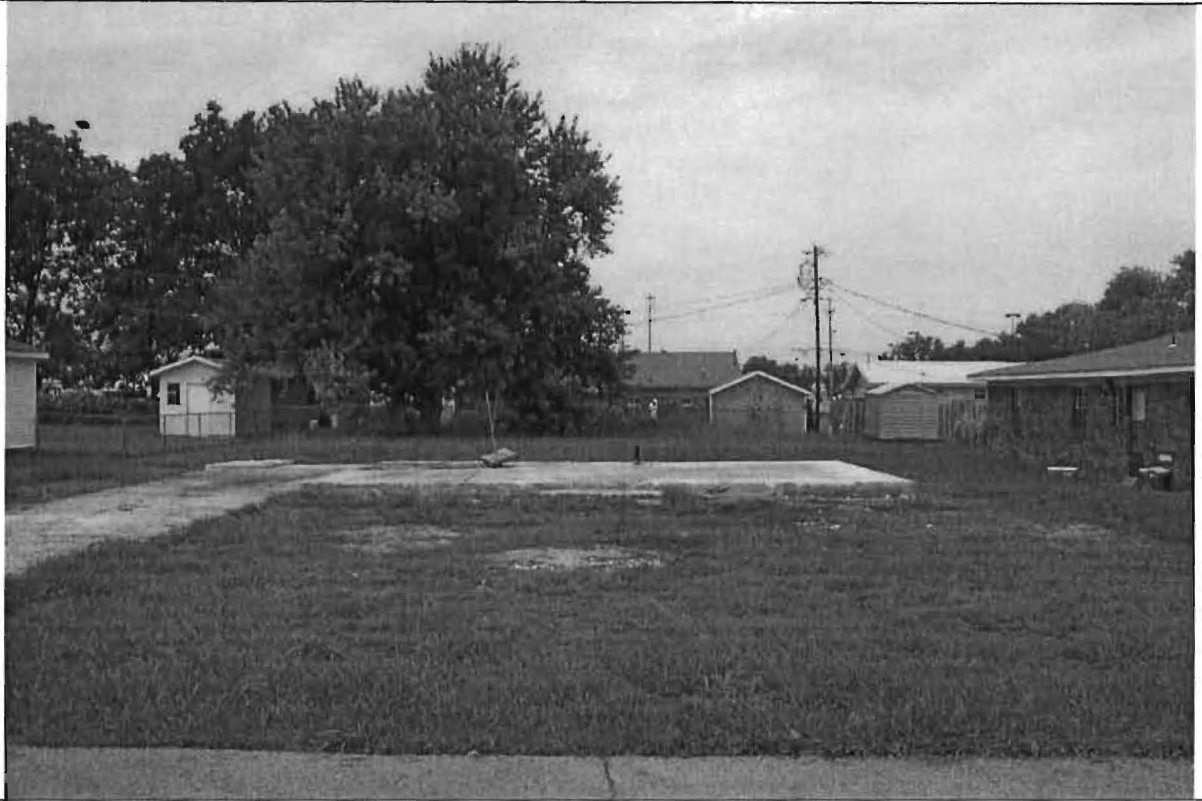
View of the site and abutting properties to the north
