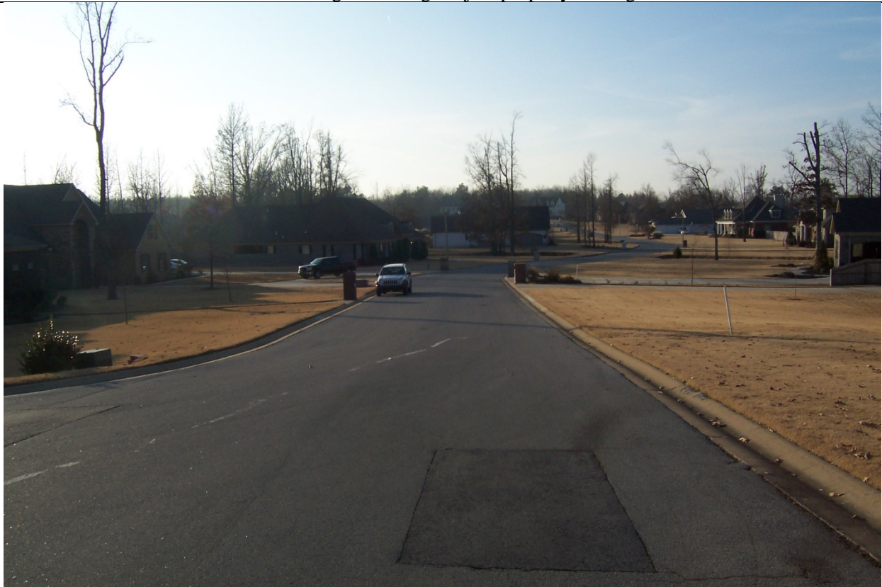
View looking west from intersection of Wolf Chase Lane/Huntcliff Dr.
