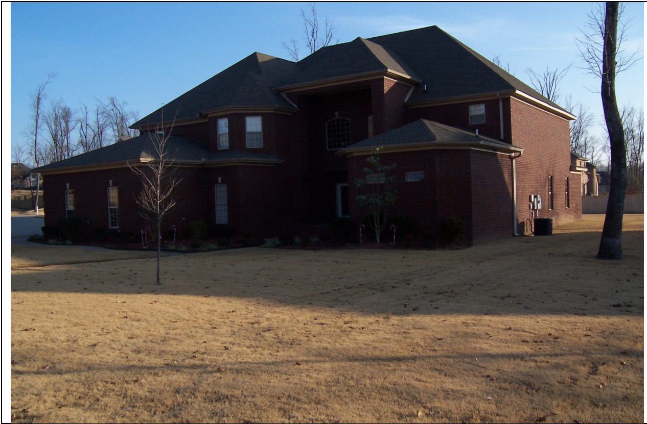
View looking south at the subject site.
