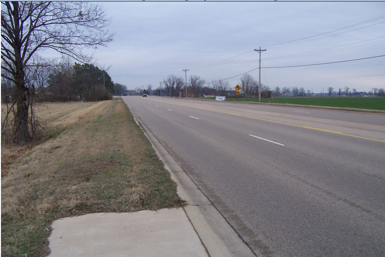
View looking East along Hwy 49S, Site to the left
