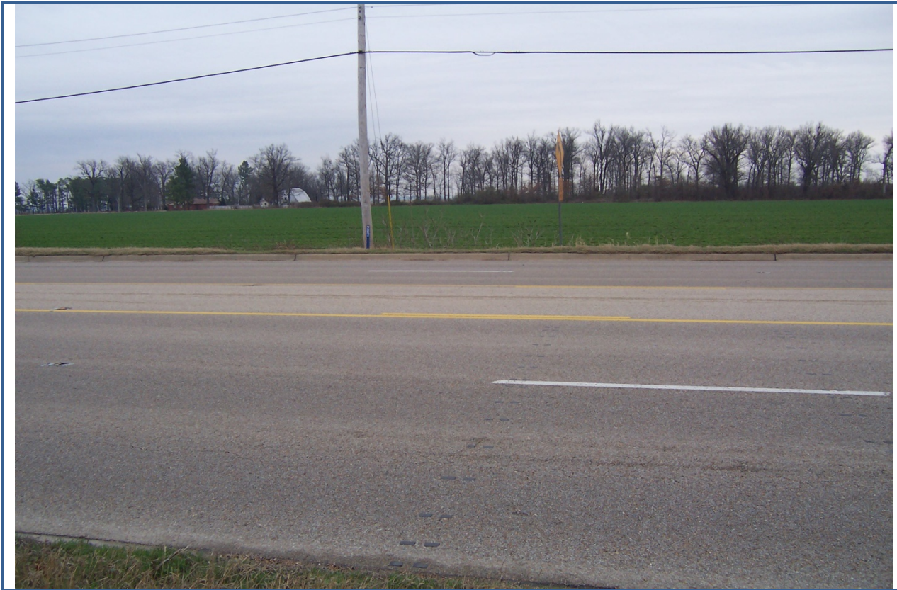
View looking South across Hwy. 49S from project Site
