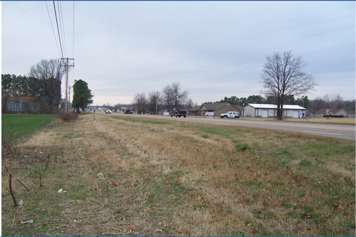
View looking West along South side of Hwy 49S, Site to the right
