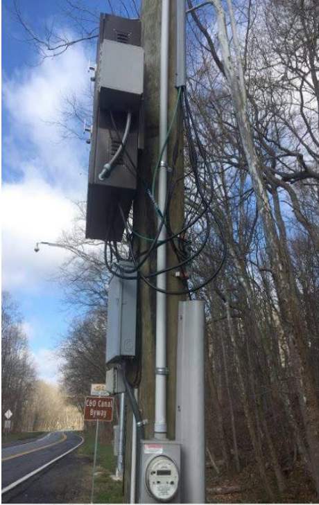
Small cellular base station equipment on "Scenic Byway" MacArthur Blvd., Potomac MD
