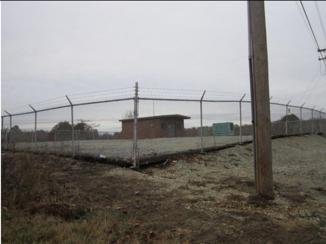
View looking east towards a CWL Power Station directly northeast of site along Hwy. 351
