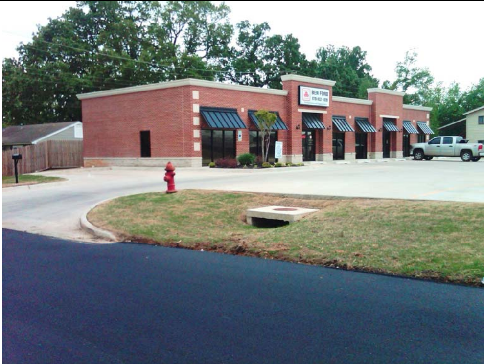
View looking Existing Site from Stadium Dr./Parkwood
