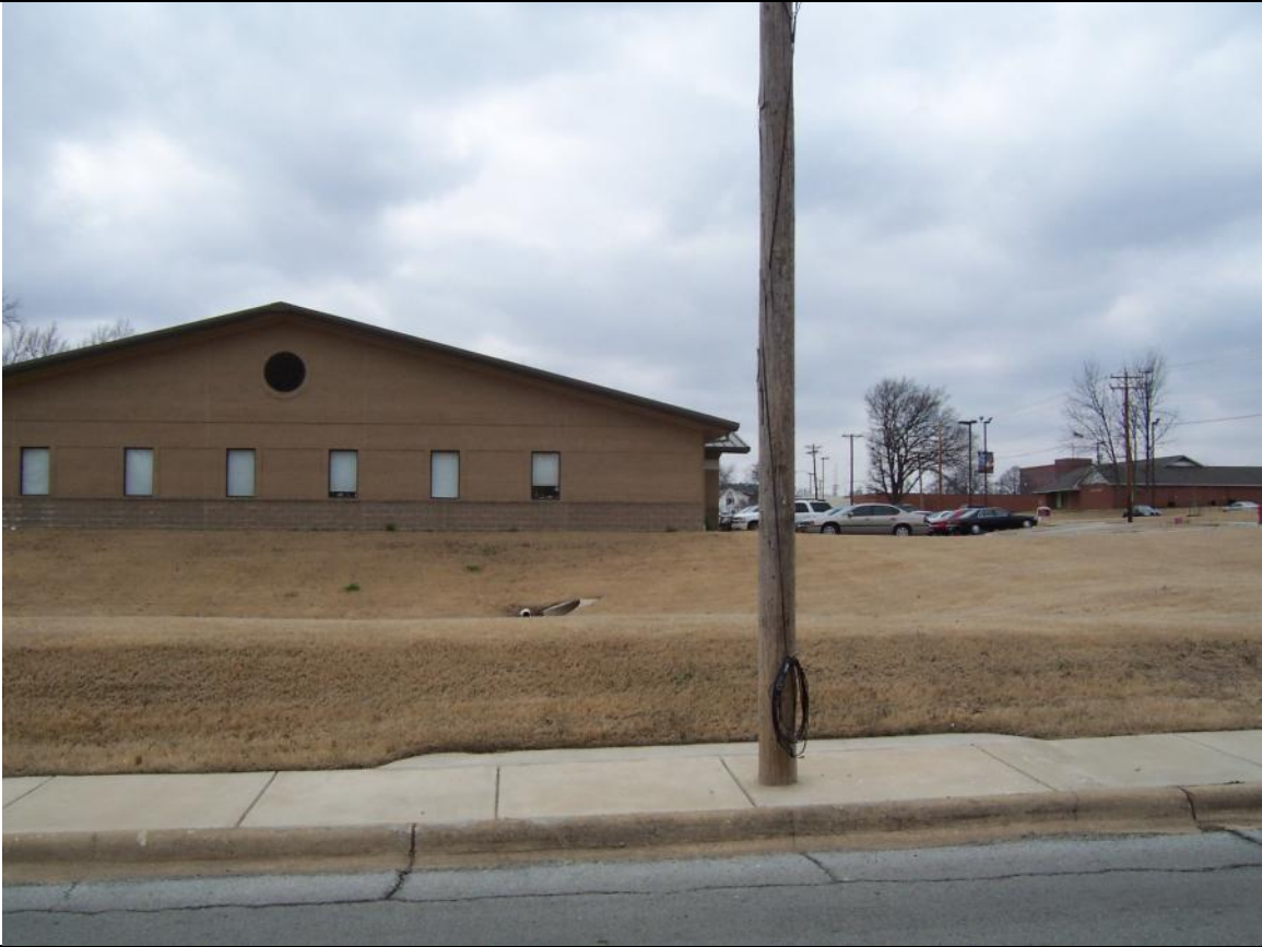
View looking West from subject site
