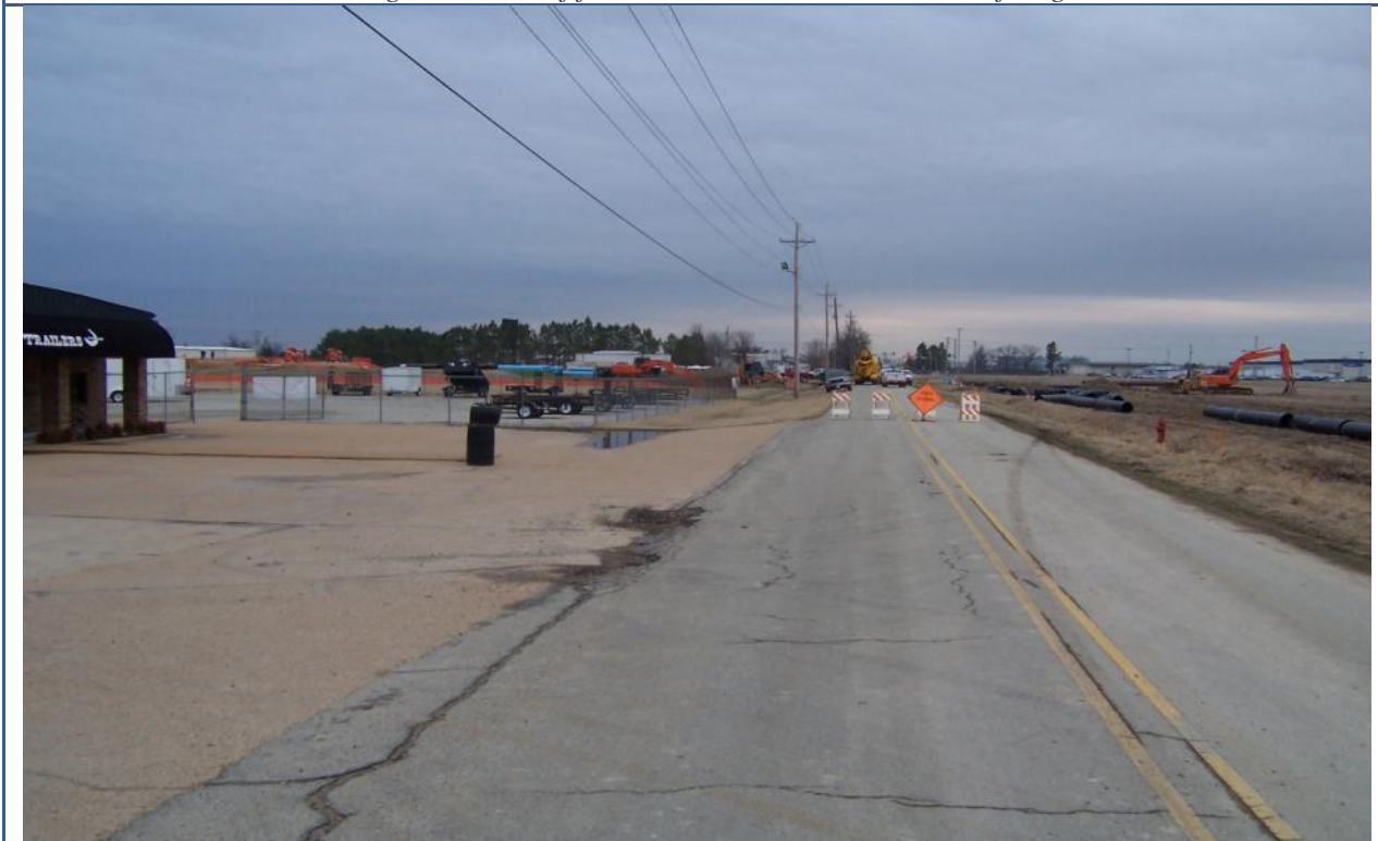
View Looking South along Commerce Rd. (CWL - installing new lines).
