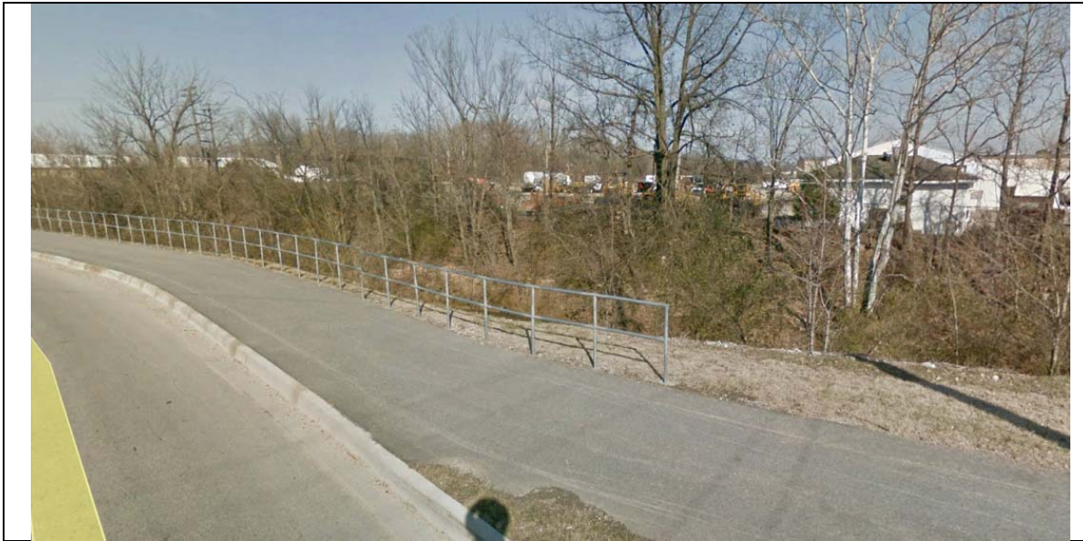
View looking East
