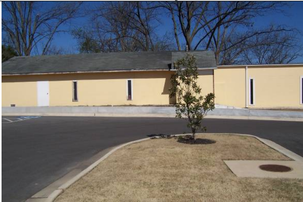
View of Site looking East
