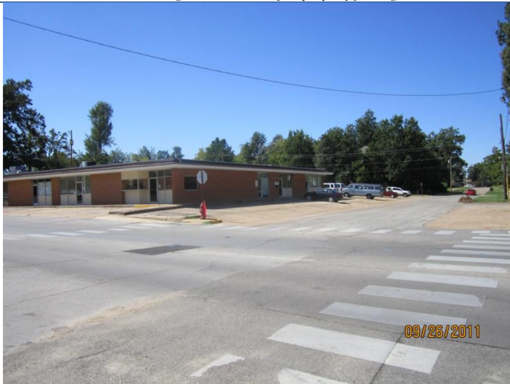
View looking West of church property.
