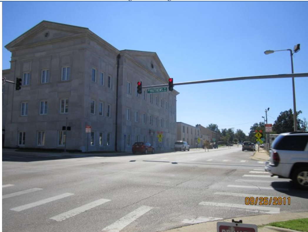
View looking South at the intersection of Matthews Ave./Union St.
