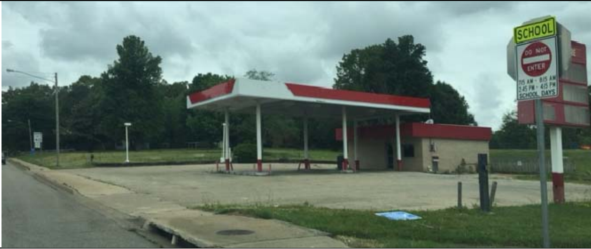
View looking west on Highland at Site
