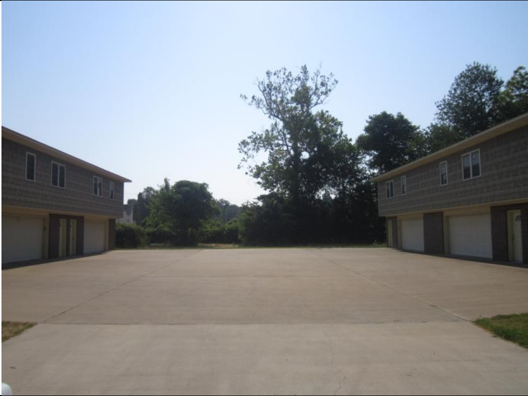
View looking East towards proposed duplex location.
