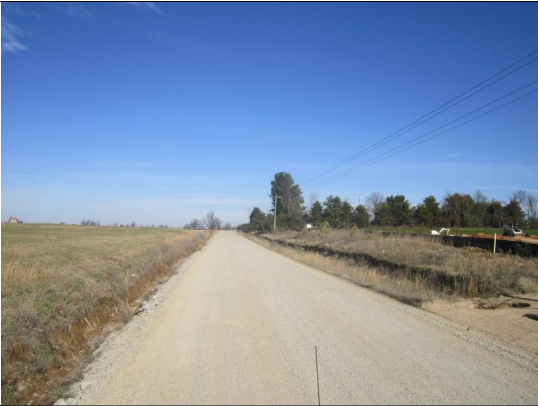
View Looking North along Clinton School Rd. (unimproved).
