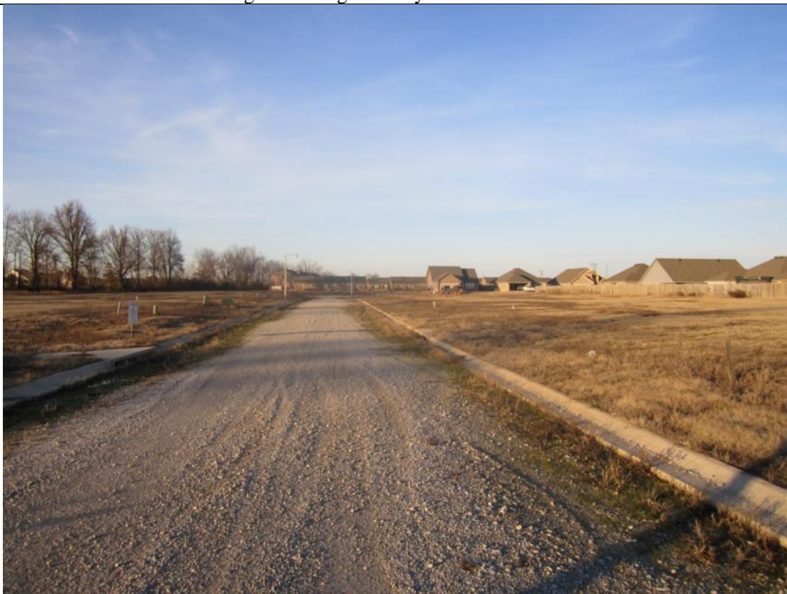
View looking North along Turfway Dr.
