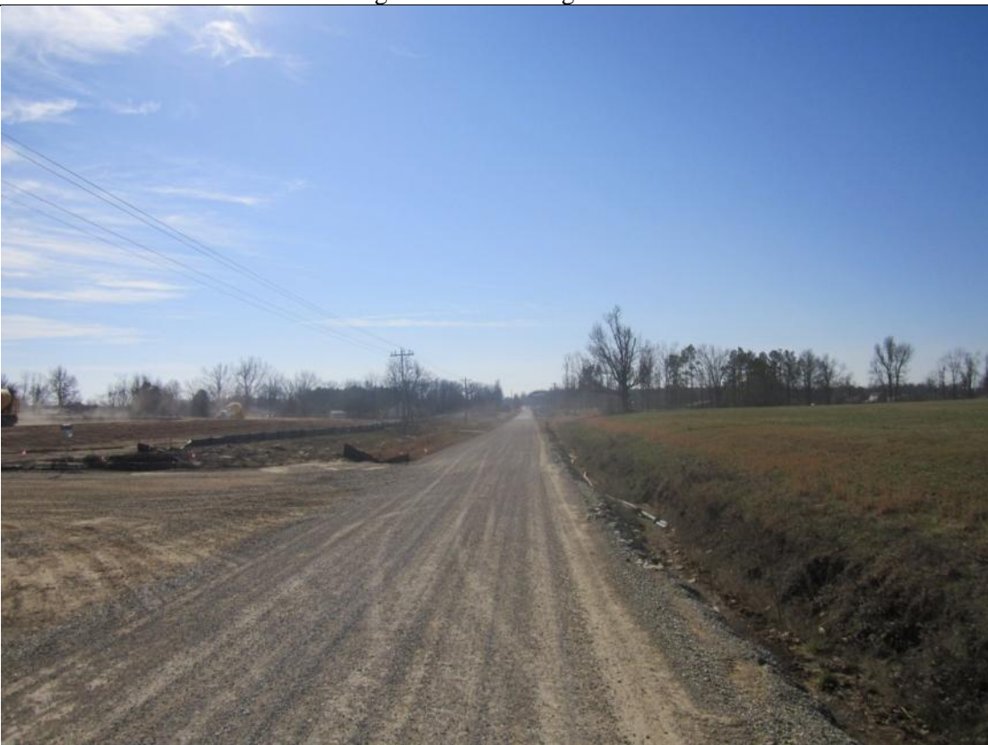
View Looking South along Clinton School Rd. (unimproved).
