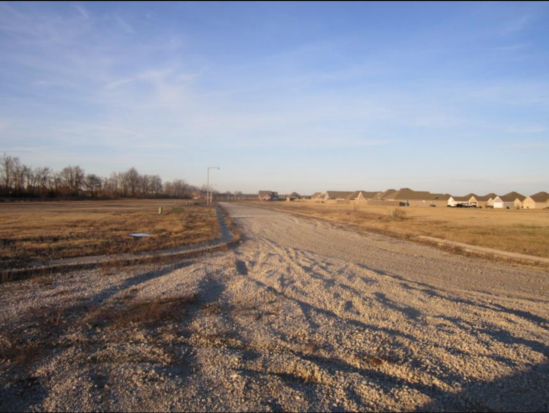
View looking North along Turfway Dr.
