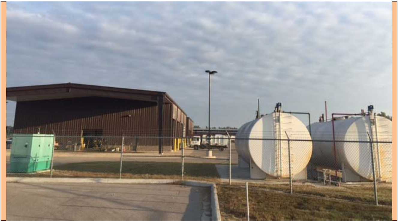
View looking North on Current Public Works Facility Location
