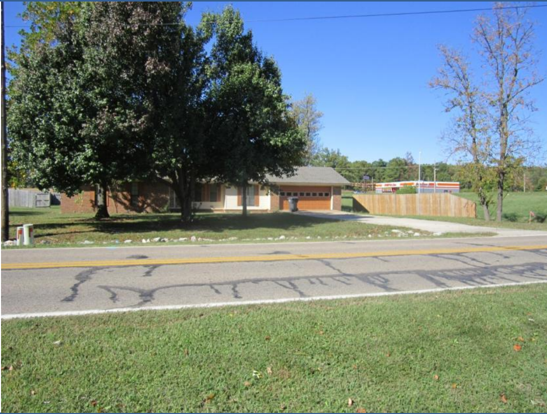
View looking West of subject property (1705 Airport Rd.)
