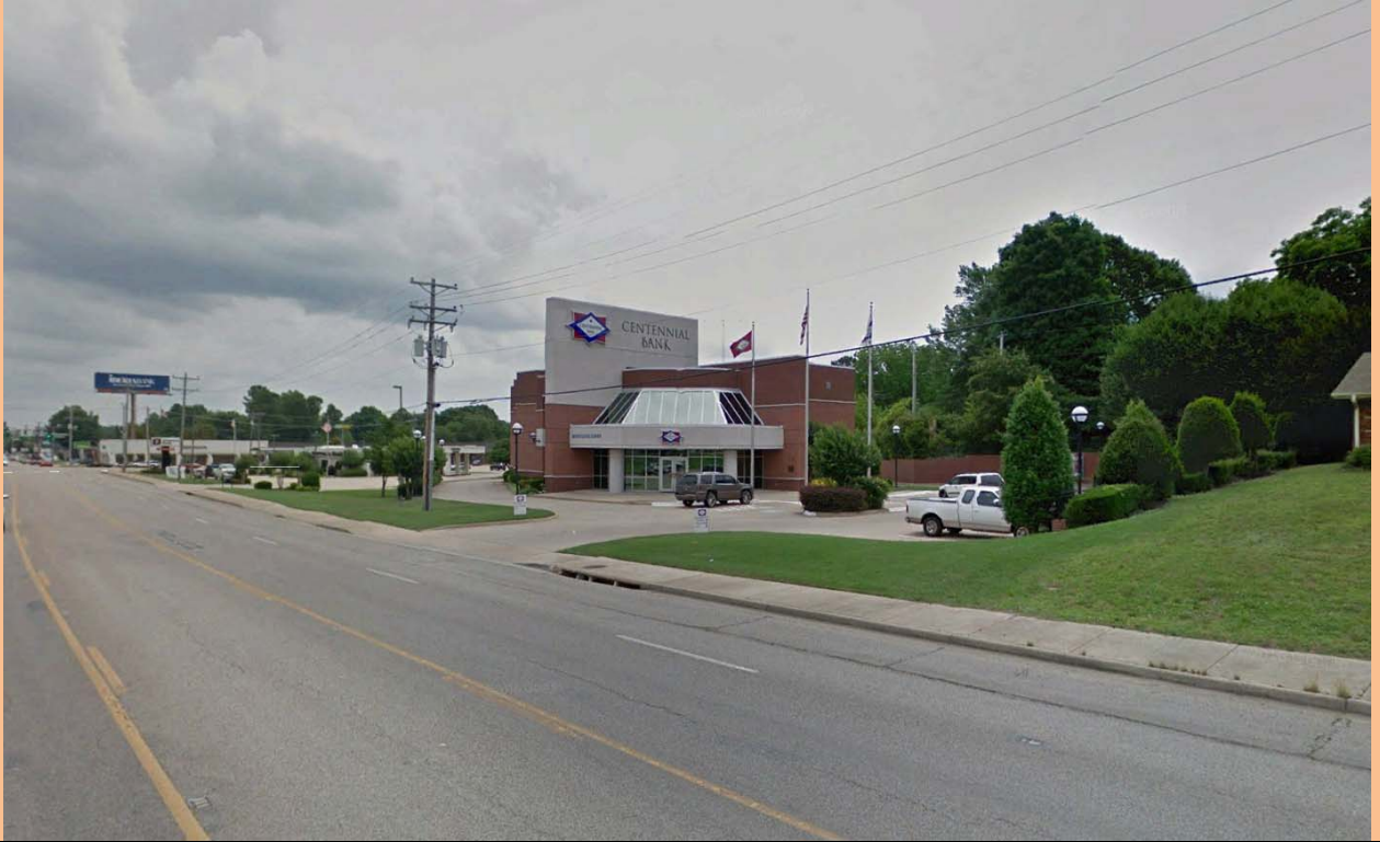
View looking East
