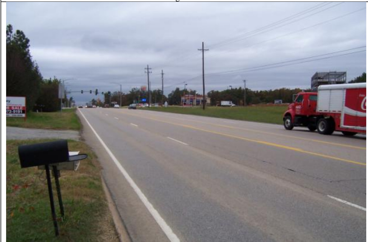
View looking southwest along Johnson Ave.
