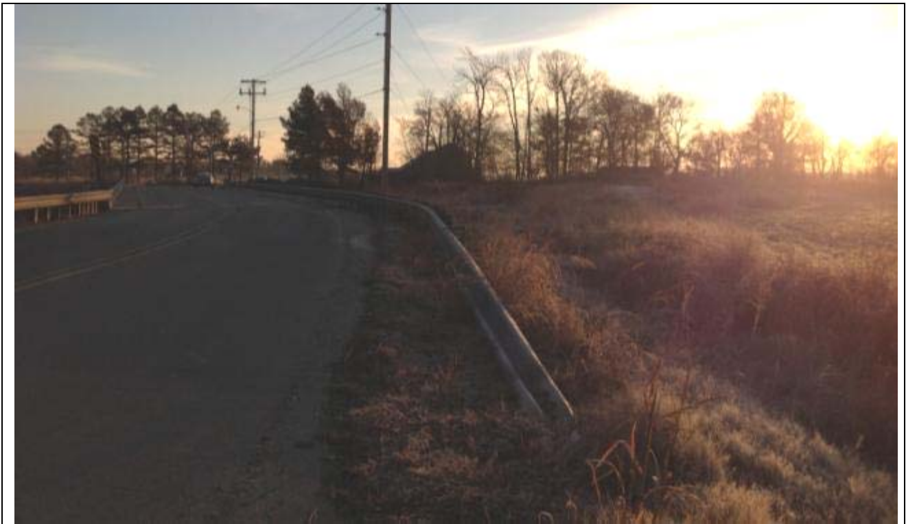
View looking East along Ingels Rd. towards the Higginbottom bridge – Project site to the right of Photo
