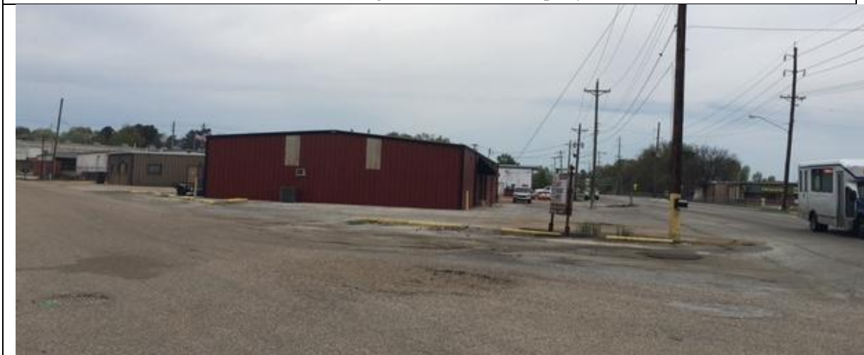
View looking North towards Property
