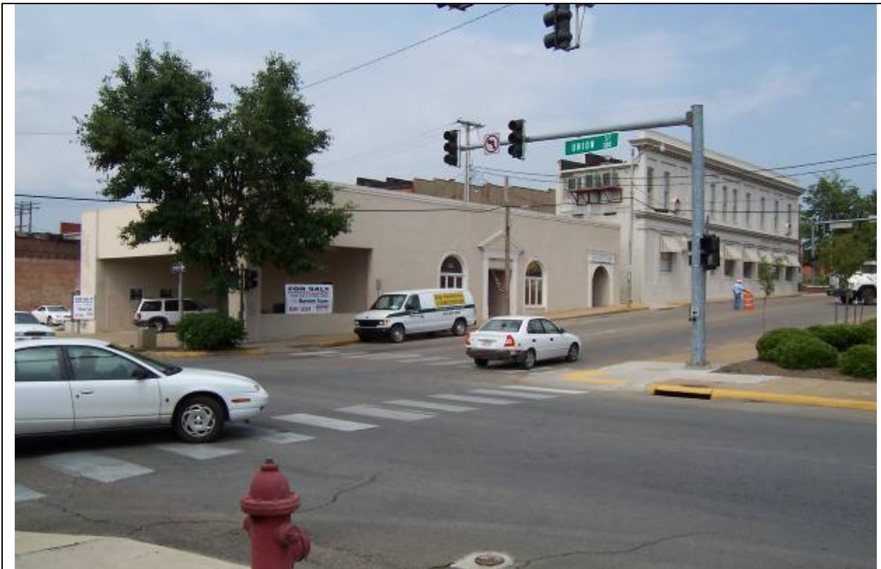
View Looking Northeast along (Huntington @ Union) intersection/frontage of project location
