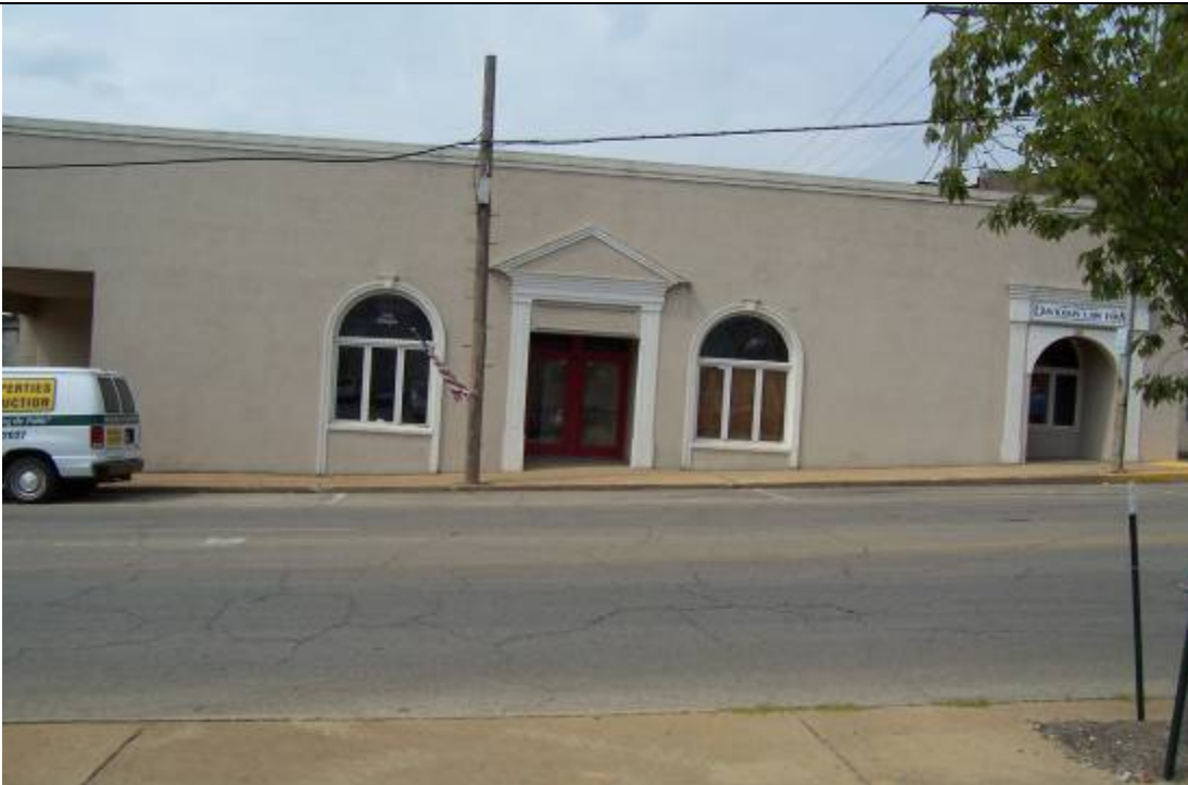
View Looking North along (Main St.) frontage of project location
