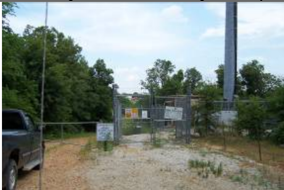
View looking North at Entrance/Casey Springs
