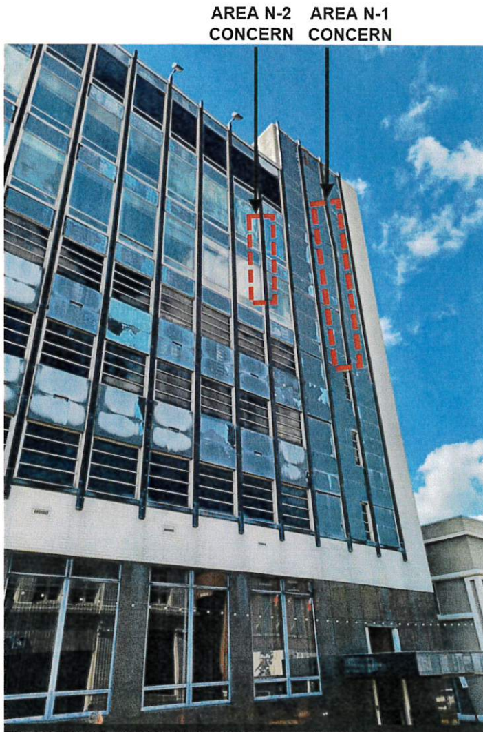
Photo 1: East Wall Elevation Showing Deflecting Wall
