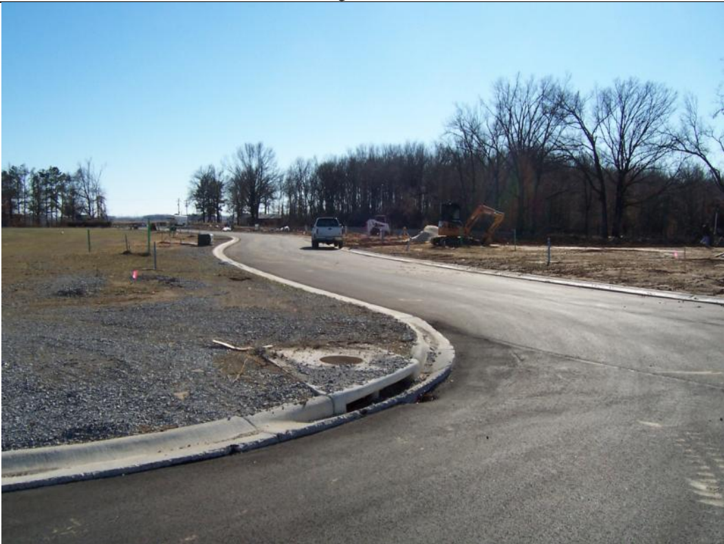
View Looking south
