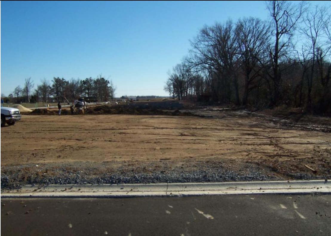
View Looking South
