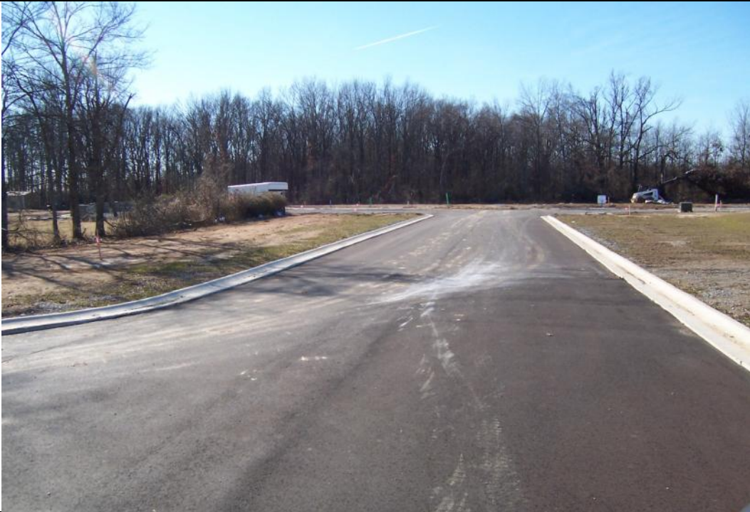
View Looking West toward site
