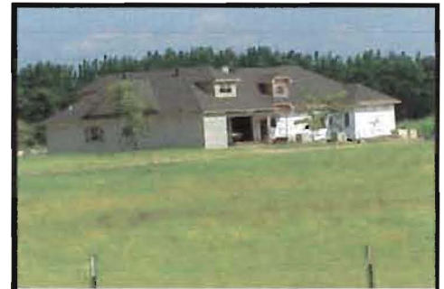
5,800 sf - 20 Acres UNDER CONSTRUCTION
