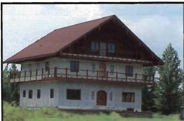
7,000 sf - 12 Acres UNDER CONSTRUCTION
