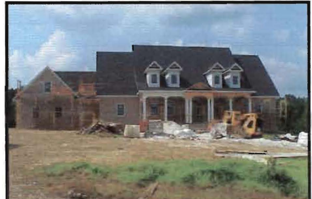
10,000 sf - 5 Acres UNDER CONSTRUCTION
