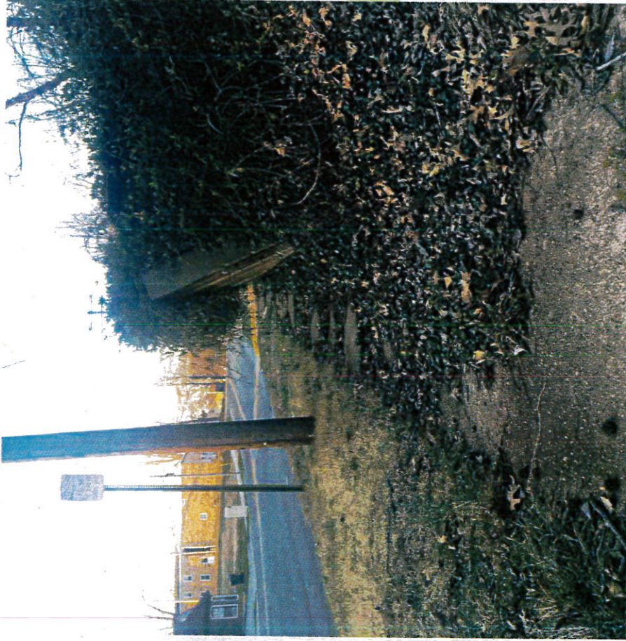
Retaining wall leaned over, impeding sidewalk near JHS.
