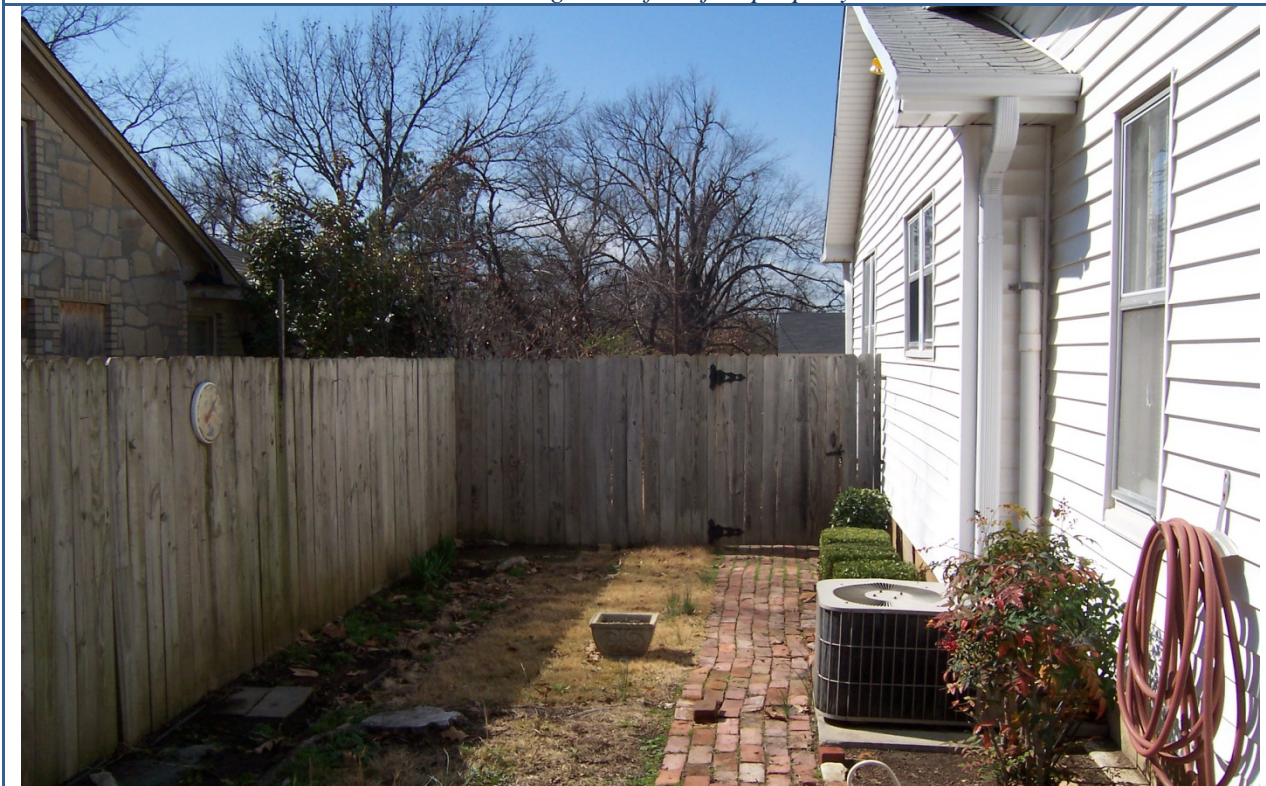
View looking West from rear yard of the side yard..
