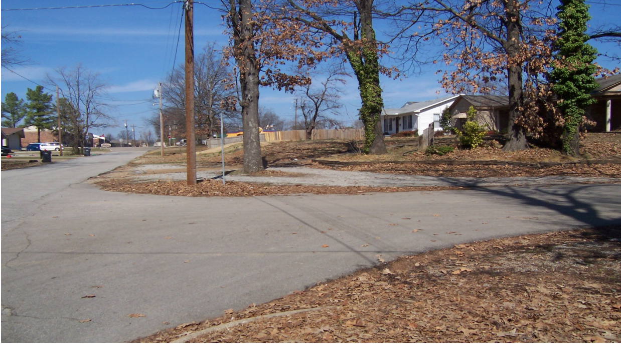
View looking North along Melrose St.
