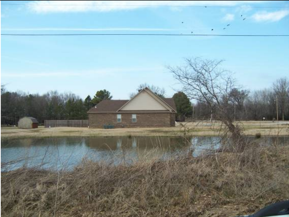
View Looking North at the property site
