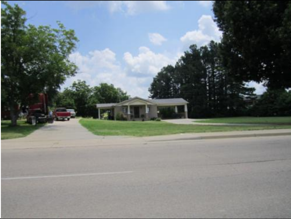
2806 North Church Street located north of site.
