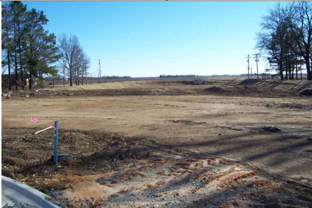
View Looking South towards detention pond
