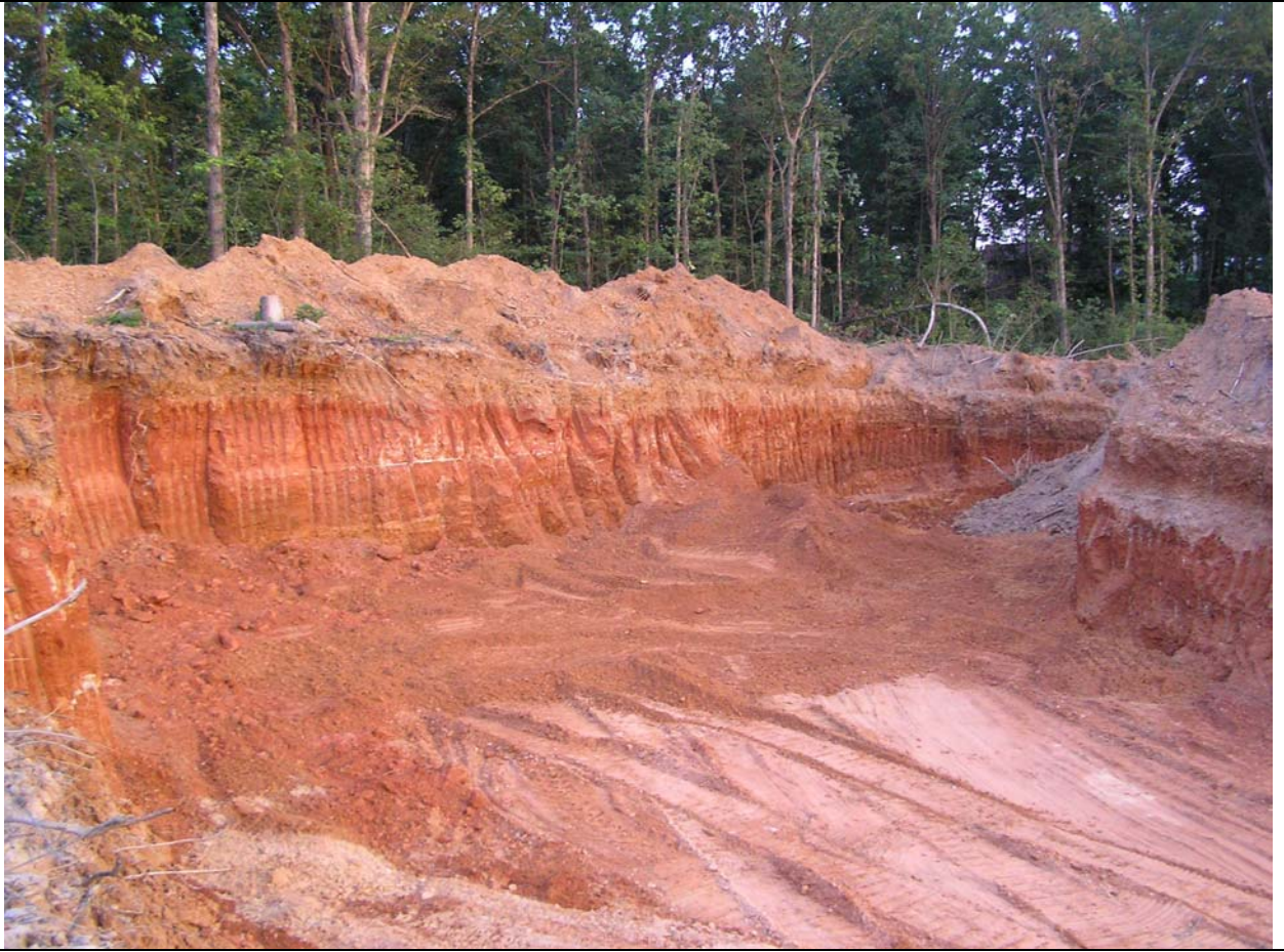
View on property site
