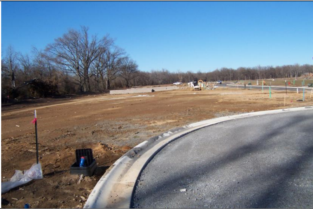
View looking north
