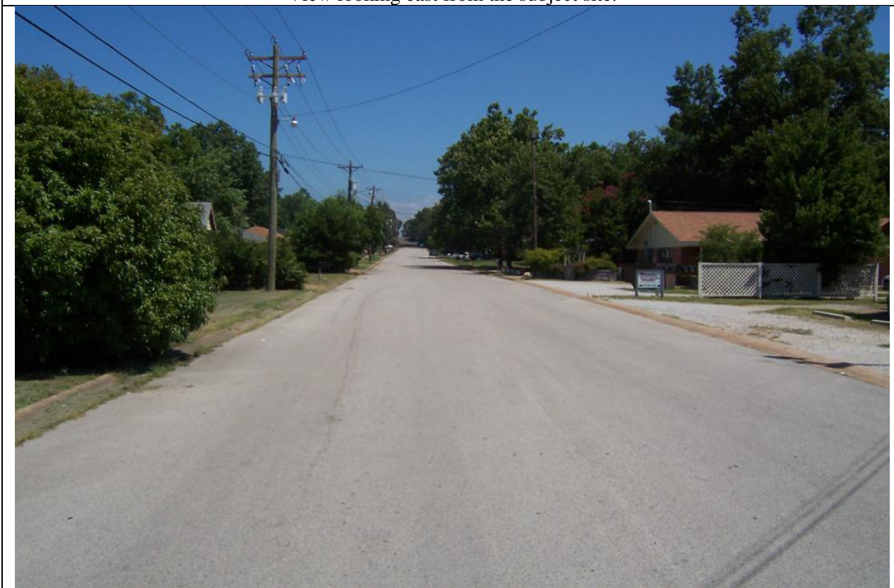
View looking north of Pardew St. along subject site.
